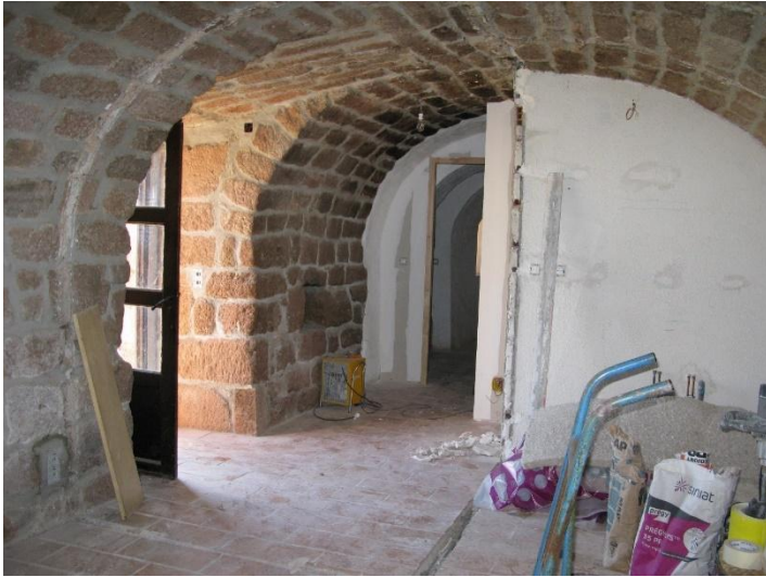
2016 : Restoration of STUDIO 4 looking north
